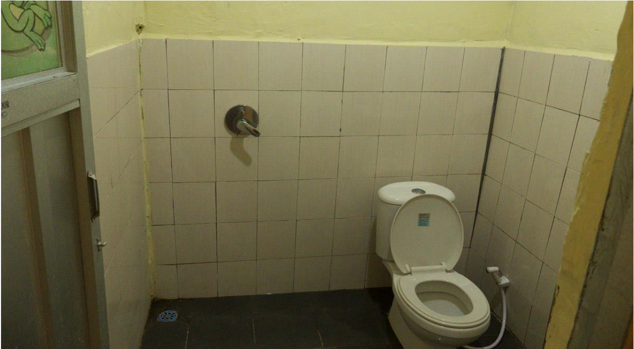
Fig. 8. A FX72 toilet from hell: no ventilation, wet crumbling concrete, metal door and mold, in the ceiling, in particular. Every surface was damp.
