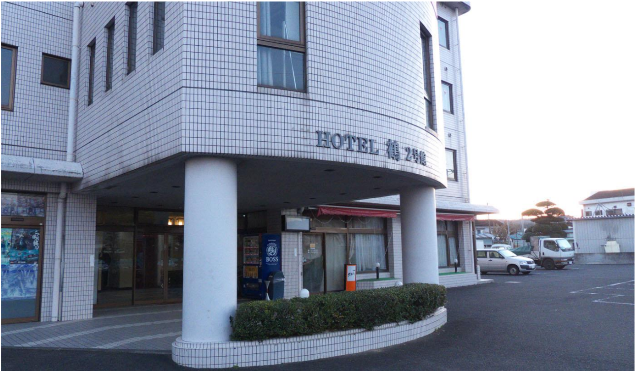
Fig. 2. Hotel Tsuru entrance, with drink vending machine and plenty of parking space. The white building on the right has a large 7/24 Family Mart.
