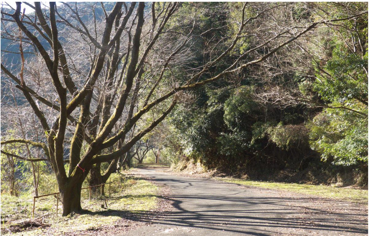
Fig. 27. The Kogawa Dam road, tarmac all the way except at a road construction site in Dec 2014.
