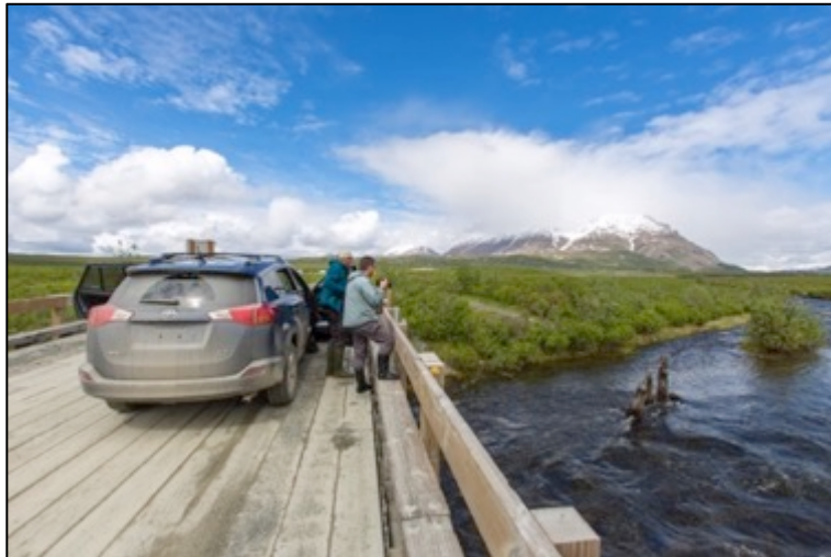
Rock Creek, Denali Highway (SC)
