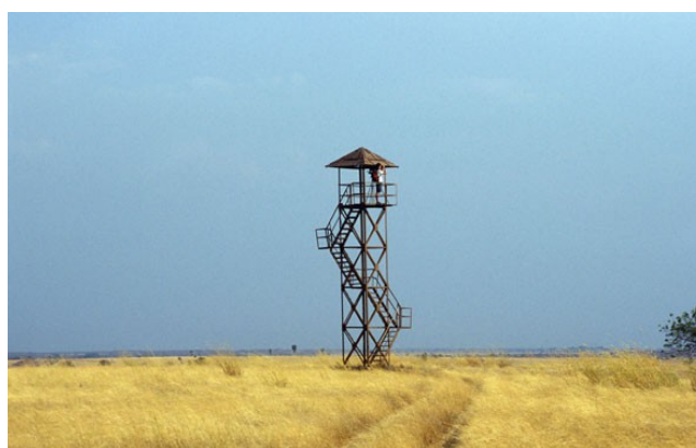
Observation-tower at Rollapadu, from where the Lesser Florican was first found, scoped very distantly.
