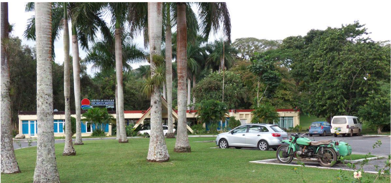
Fig. 13. The reception building of Hotel Villa Soroa.
