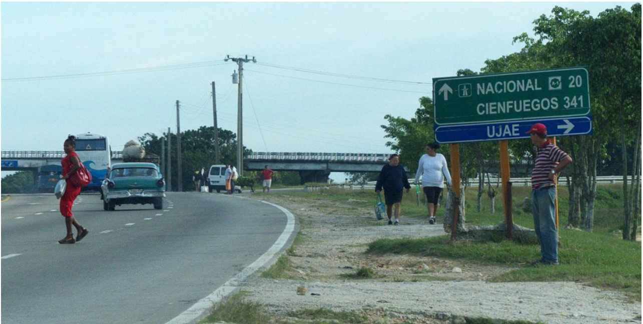
Fig. 8. The Ujae ramp, at the end of Pinar del Río Highway, a starting point of the Havana bypass.
